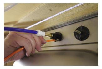
5. Now push the supplied piece of 3/8" black tubing on the larger brass barb on the bottom of the faucet. Be sure the tube is completely pushed on the barb or a leak could occur.
