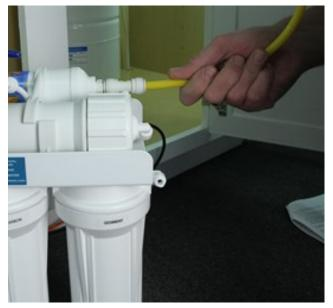
3. Connect orange tubing from the angle stop supply valve to RO unit at the sediment filter inlet fitting.
