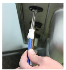
4. If an air gap faucet is being used continue to the next steps. Push the 1/4" drain line from the RO module on to the smaller brass barb on the bottom of the faucet. Be sure the tube is completely pushed on the barb or a leak could occur.
