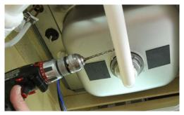
2. Drill 1/4" hole at mark through one side of pipe. CAREFUL not to drill through both sides of the pipe.
