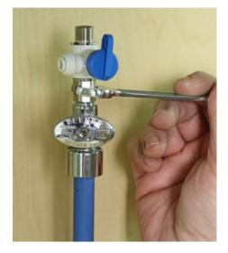
2. Now install the whip hose or tubing on the angle stop valve and tighten.
