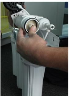
5. Lubricate the O-ring on the membrane housing and install H. RO unit installation the cap hand tight. Tighten the cap an additional 1/8 - 1/4 turn.
