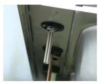
Once the faucet is secure, install the 7/16" UNS x 3/8" QC faucet connector on the threaded nipple. This fitting doesn't require sealant. This fitting will seal at the beveled surface. Tighten the fitting hand tight then an additional <sup>1</sup>/<sub>2</sub> turn with a wrench or pliers.
