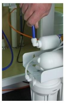
2. BE SURE the storage tank shutoff valve is in the Permeate Pump Installation attached to the storage tank. Connect the open end of the green tubing from tank to RO unit at the post carbon filter inlet tee fitting. Leave the tank valve closed.
