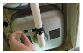
3. Position both halves of drain saddle on drain pipe so threaded opening lines with hole. A screwdriver may be used to keep the holes oriented during the tightening process.
